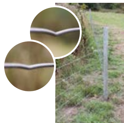
Step 6 Finally tension fence to allow tension curves to reduce by 50%, Job done!
