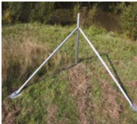
Step 1 Secure your corner/end strainer
