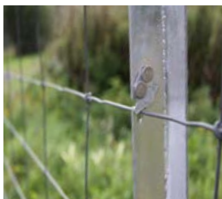
Step 5 Push the wire down, the keeper will automatically close
