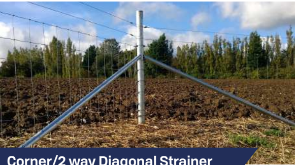
Corner/2 way Diagonal Strainer
