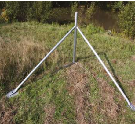
Step 1 Secure your corner/end strainer
