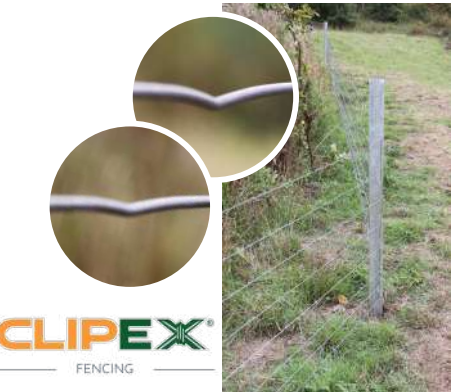
Step 6 Finally tension fence to allow tension curves to reduce by 50%, Job done!
