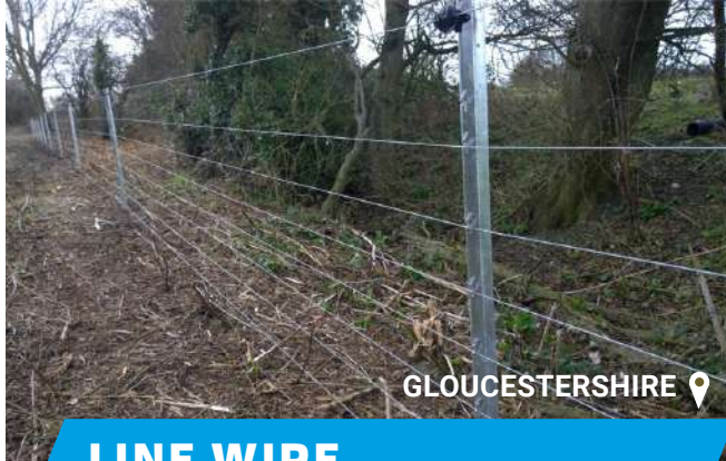
LINE WIRE FLOOD FENCE
