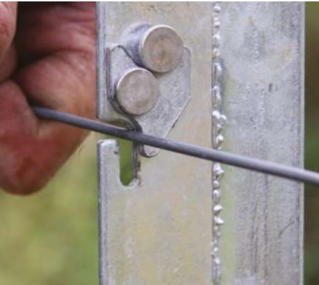
Step 4 Push the wire into the slot putting pressure on the keeper
