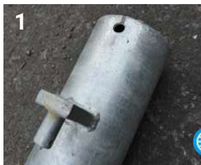
1 An inverted top hinge to prevent easy gate removal
