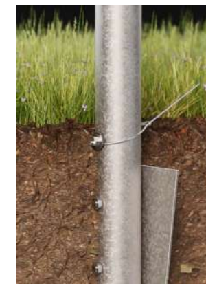
7. Screw in and tie off bottom of GRIPPLE GPAK.
